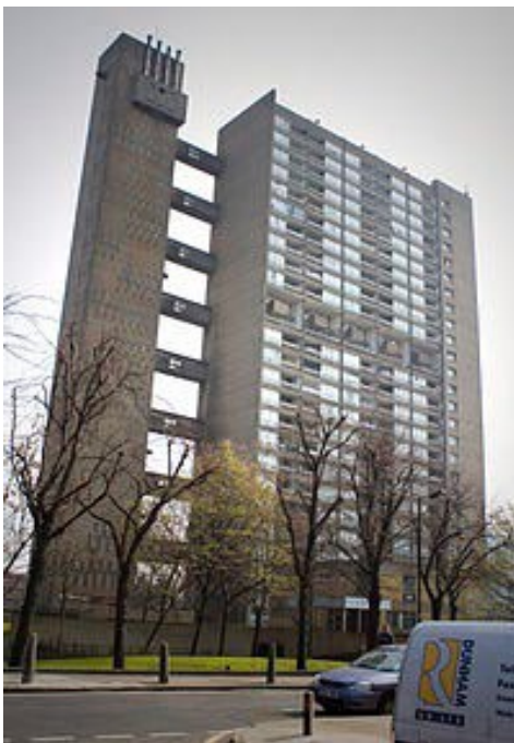
Figure 1 Balfron Tower, Poplar, a Grade II* listed tower block designed by Erno Goldfinger in 1963 for the London County Council, built 1965–1967, which adopts the same separated circulation tower as Aquarius. (Source: Wikimedia)
